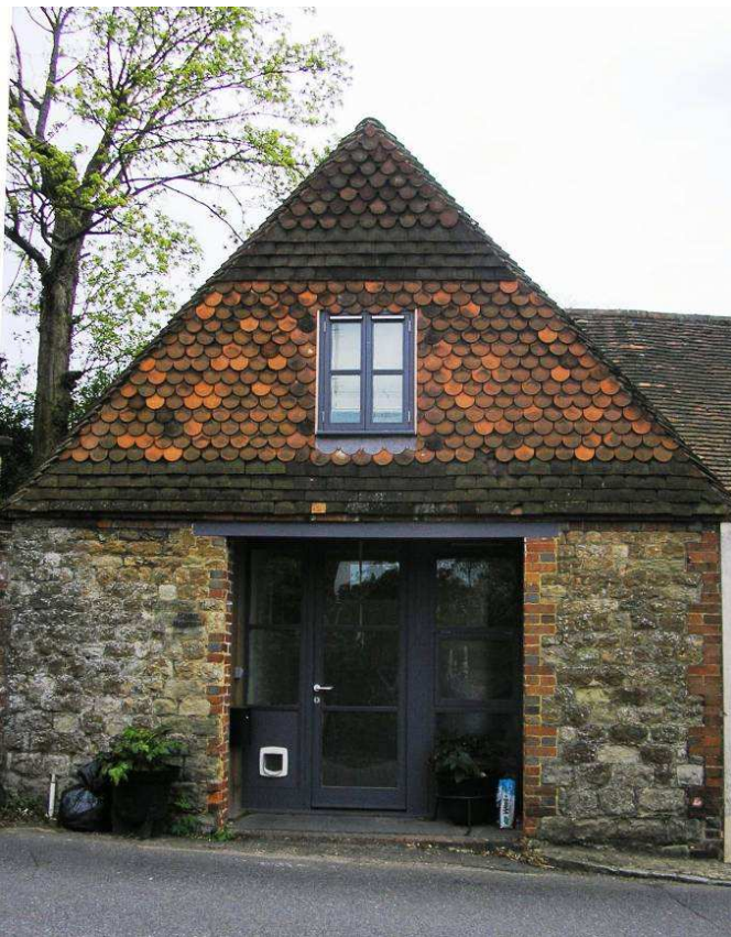
A simple modern conversion retaining original character
