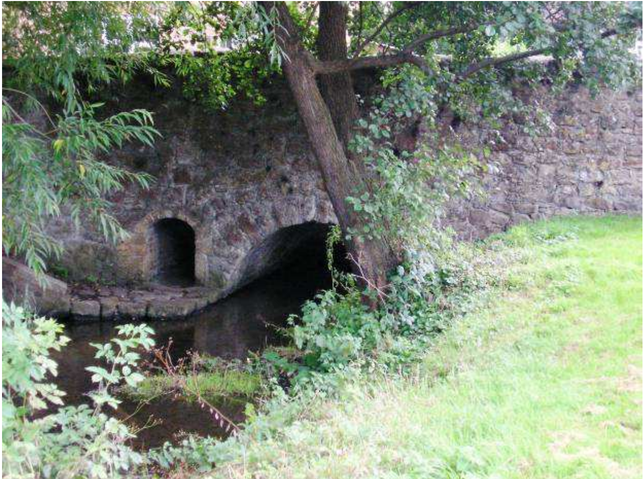
Historic ragstone bridge
